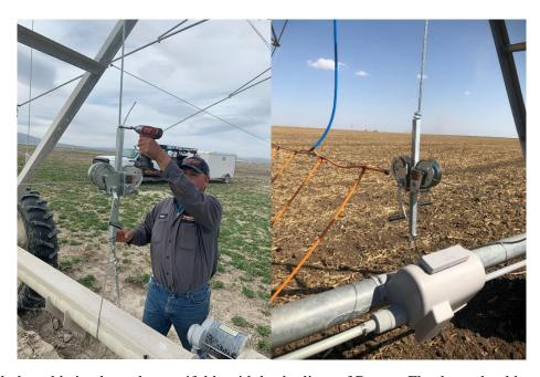
Step 6: With the cable in place, the manifolds with leader lines of Dragon Flex hose should now be unrolled and attached to the cable. Hang the manifolds to the cable loosely with wire or other device to allow for easier handling. Using the wire ties provided manifold should be tied to the cable at each tee and each adaptor tee used to feed water to manifold. Wire ties should wrap around the cable at least two to
